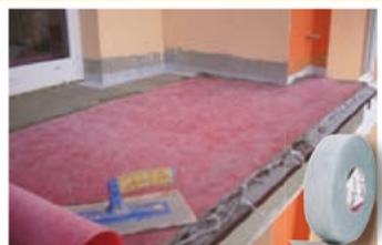
SELF-ADHESIVE SEALING TAPE may also be used
