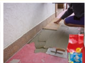
Apply DLAŽBULEP mortar and install tiles
