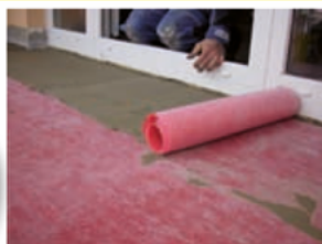
Install in a layer of adhesive and overlap the seams by 10 cm
